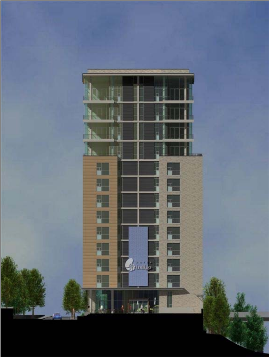
East End Of Building – Main Lobby Entry
