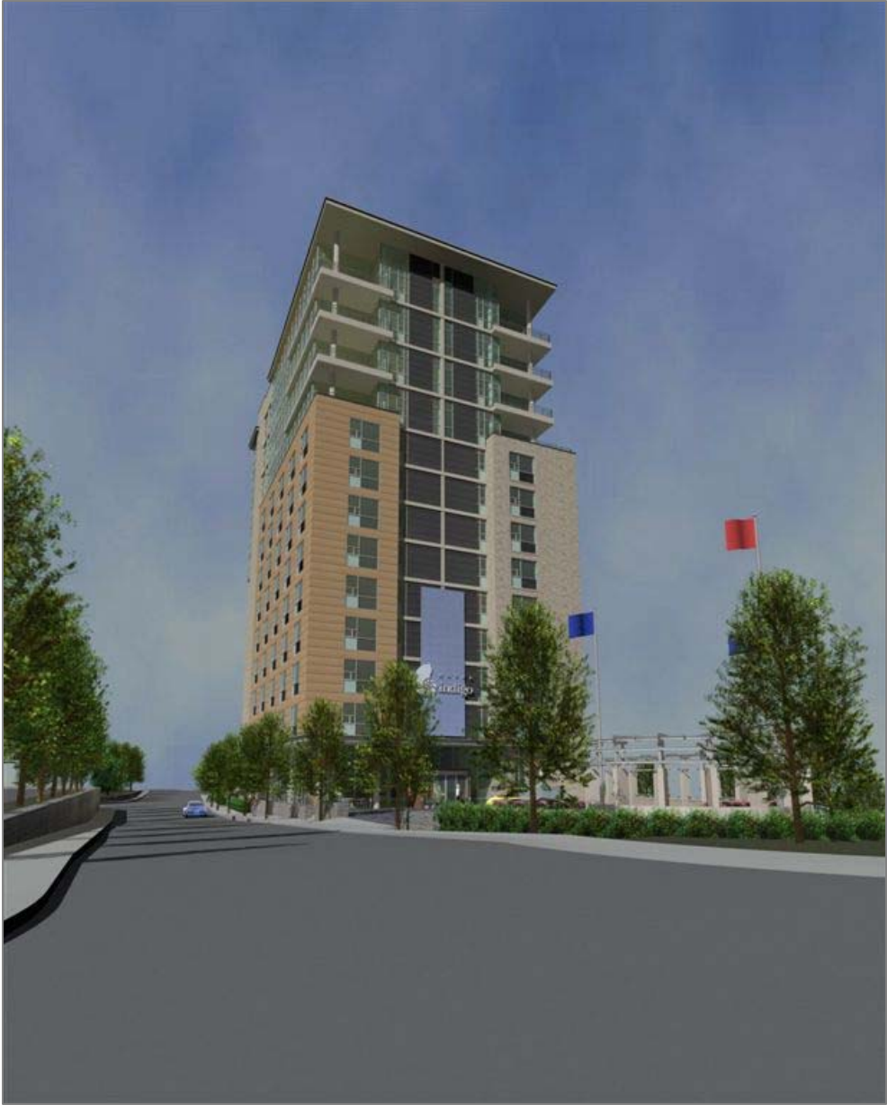
Looking West On Haywood Street
